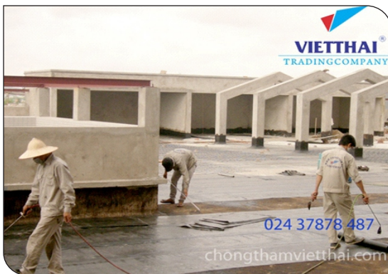
Construction of torched on membrane
